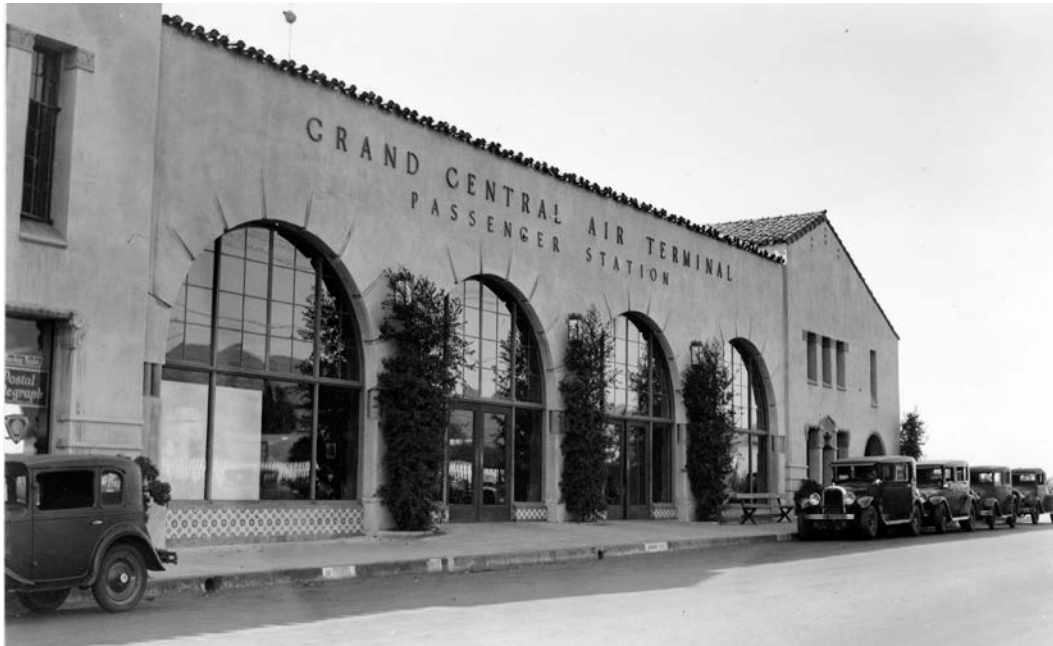
Figure 16 Exterior, north façade, view looking southwest, 1937 Source: Bison Archives
