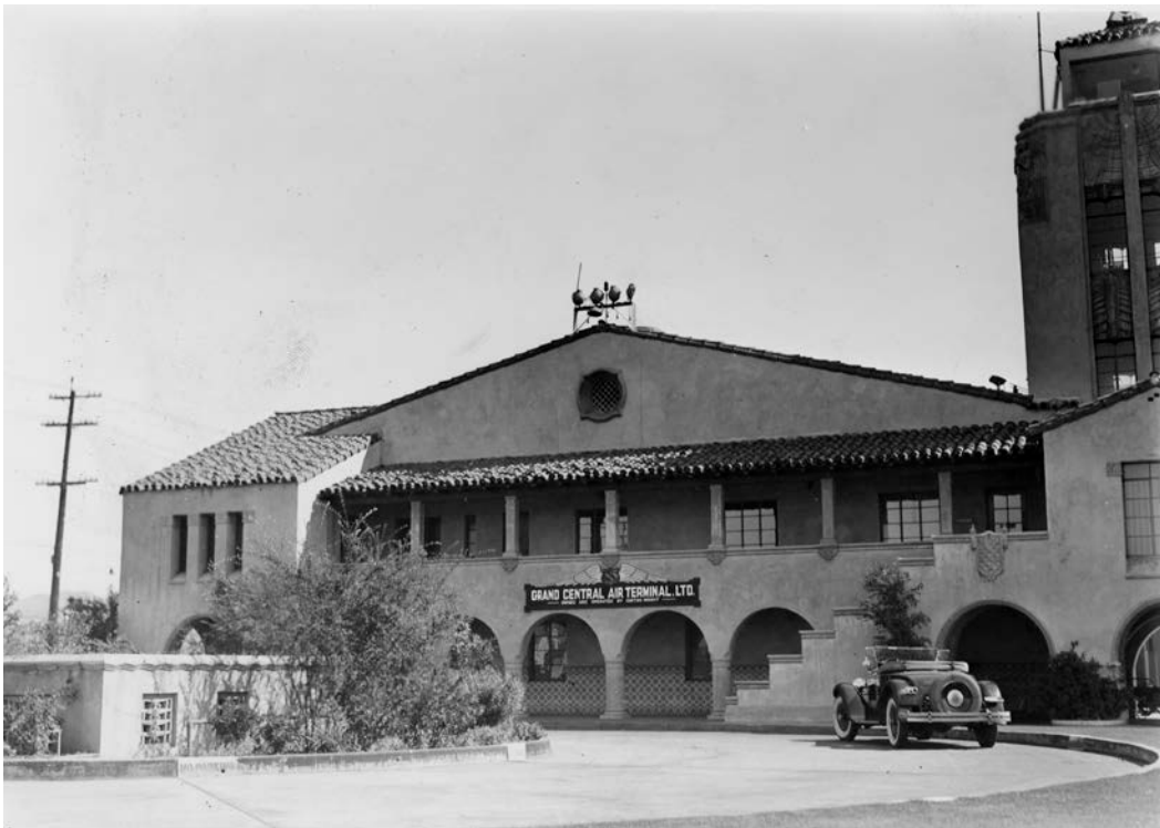
Figure 17 Exterior, west façade, circular drive and vault, view looking northeast, 1937 Source: Bison Archives
