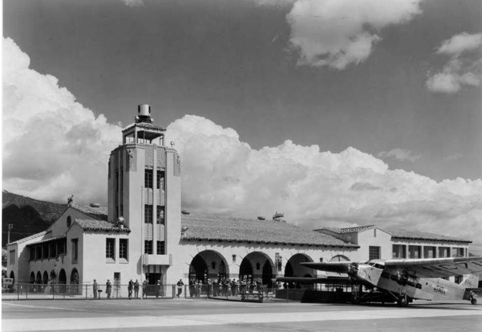
Figure 8 Exterior, south façade, view looking northeast, c. 1930 Source: California State Library Archives
