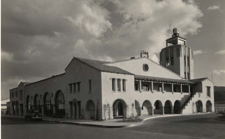
Figure 6 Exterior, north and west façades, view looking southeast, c. 1930 Source: California State Library Archives
